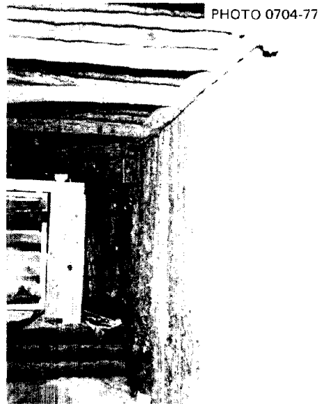
Fig. 4.7. Small-Pole Shelter after being tested with blast doors closed at the 53-psi overpressure range. Note the slightly damaged expedient shelter ventilating pump in the stoop-in entryway. Two men worked about 5 min to replace the four blown-loose flaps, the only damage.
